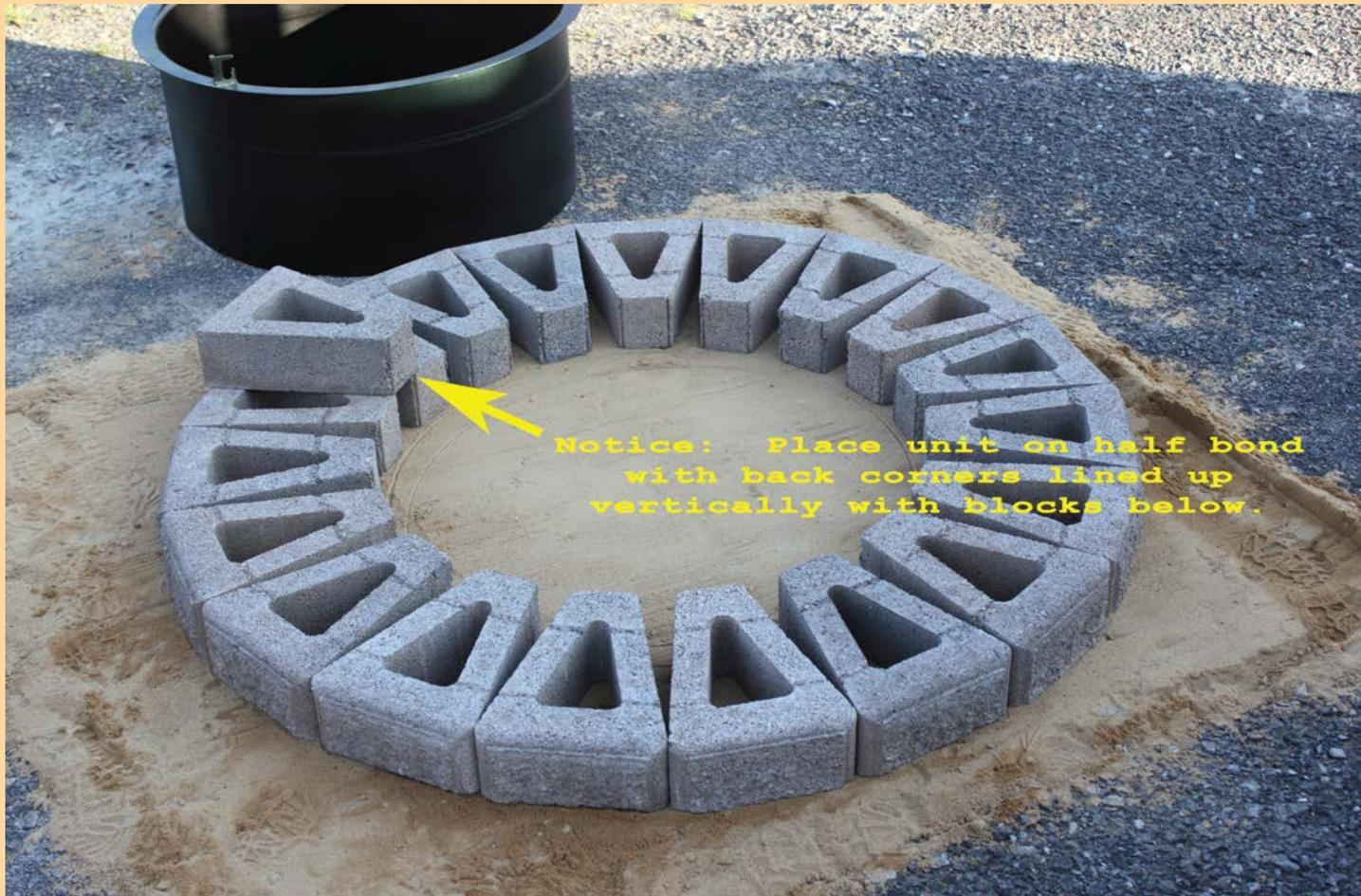
**It is recommended to use construction adhesive between blocks!**
